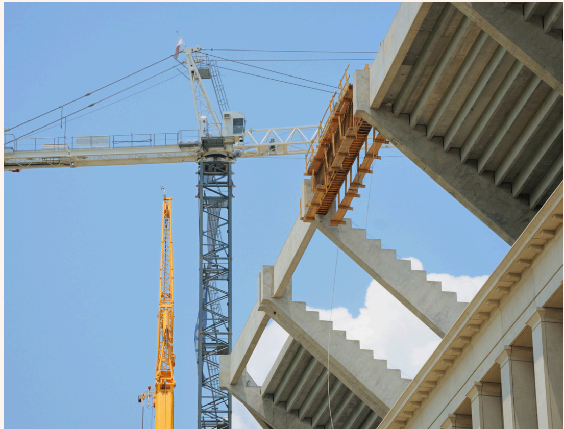
Construction continues on the new Colossal stadium, a centerpiece of Piccadilly’s 2028 Colossal Games preparations
